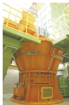
Pulverizer for non-burnable wastes
