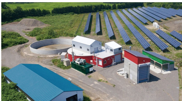
Bio gas plant
