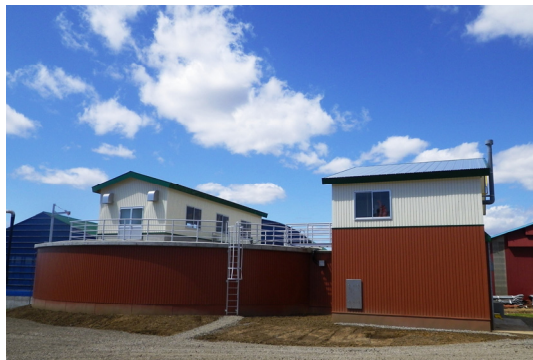
Bio gas plant
