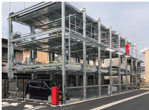
Mechanical multistory parking equipment
