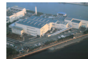
Non-burnable waste recovery facilities
