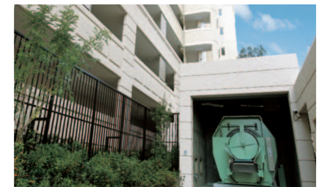
Drum-type waste storage and discharge equipment
