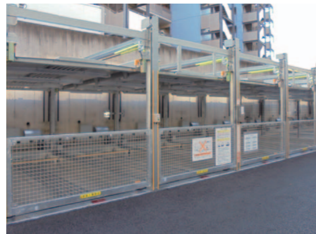
Mechanical multistory parking equipment
