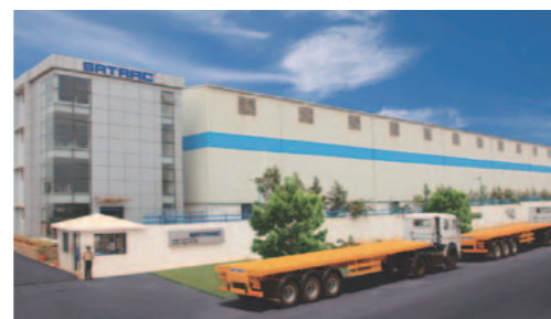
SATRAC ENGINEERING PRIVATE LIMITED Occupies : 24,292m 2
