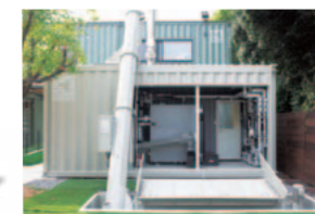
Wood biomass boiler unit
