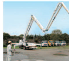
Operation test of the boom of a concrete pump
