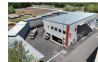
Waste transfer stations
