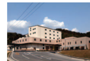
Bulky waste treatment facilities
